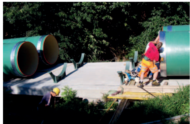
For the installation of an adapter piece
